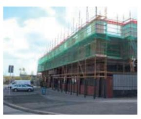
Photograph 11 Scaffold erected on a wide footway.
