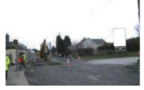
**Photograph 9** Roadway open at busy junction; available width of road reduced; no traffic management plan in place.
