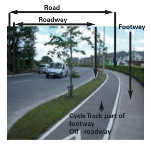
**Photograph 3** Section of road showing both that the cycle track is part of the footway and that the footway is associated with a roadway.
