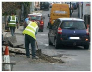
**Example 4** A worker carries out work activity with his back to oncoming traffic on the roadway. No arrangements are in place to control the movement of public vehicles close to site workers.
